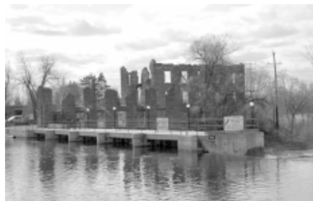
FIGURE 2 Environmentally low-impact hydro sites require careful site planning and deployment. The Appleton, Ontario Ecologo-certified plant owned by Canadian Hydro Developers is a run-of-river, 1,350 kW site comprising 2 propeller and 1 Kaplan turbine. Construction was intended to blend into the surrounding residential area by keeping the powerhouse low to the upstream view, preventing obstruction of the historic mill ruins.
