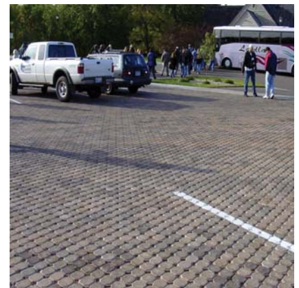
EXAMPLE OF PERMEABLE PAVING IN A PARKING LOT
