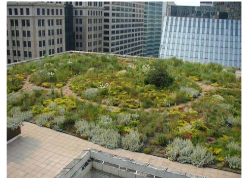
GREEN ROOFS ARE ONE URBAN HEAT ISLAND MITIGATION STRATEGY - GREEN ROOF ON CHICAGO CITY HALL.
