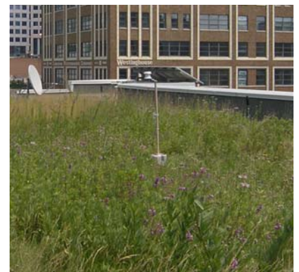
ROOF TOP AIR TEMPERATURE MONITOR, MOUNTAIN EQUIPMENT CO-OP ROOF TORONTO, JULY, 2007
